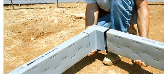
Form-A-Drain offers drainage, waterproofing and specialty solutions designed to keep foundations solid from the ground up and is made from 100% PVC scrap.
